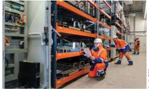
A 4.5MWh BESS using Audi EV batteries brought online by RWE in January 2022.
